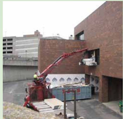
Materials delivery via window
