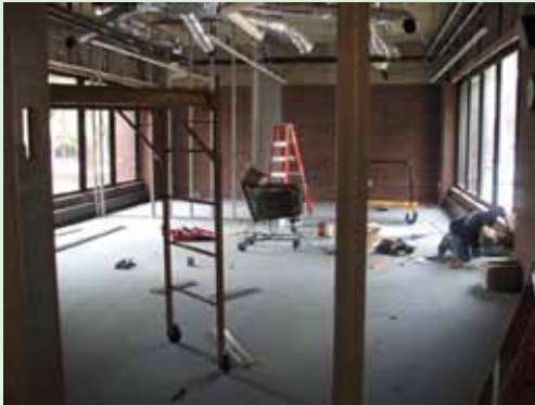
Circulation workroom in progress
