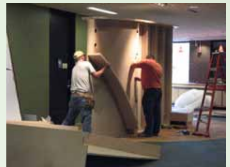
The display wall is assembled on-site
