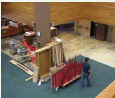
Lobby remodeling underway
